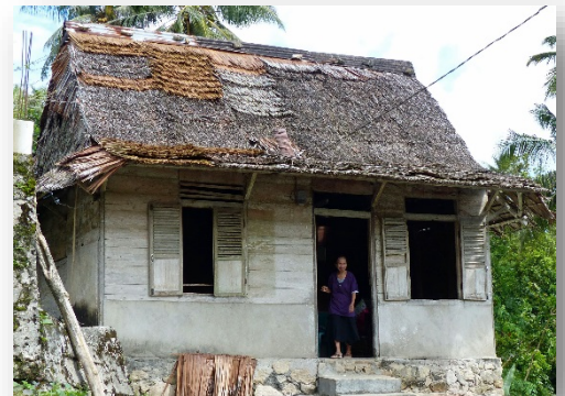
One of the homes with repaired thatch roof
